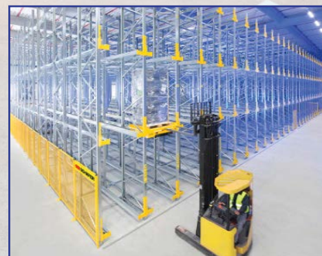
Kho sử dụng Pallet Shutter Warehouse using Pallet Shutter
